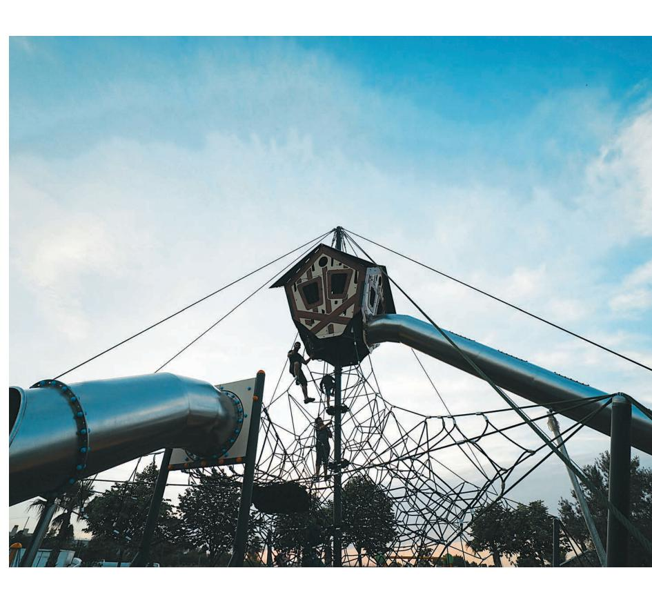
CmrRope ™ is formed by 6 strands of galvanized wires and a core either steel or fiber. Each strand is tightly braided with Polyester which is adhered to galvanized wires with a patented method to create a solid surface where polyester meets with wires. So extra protection is achieved against friction and vandalism. Surface is extremely abrasion and UV resistant also fire retardant.
